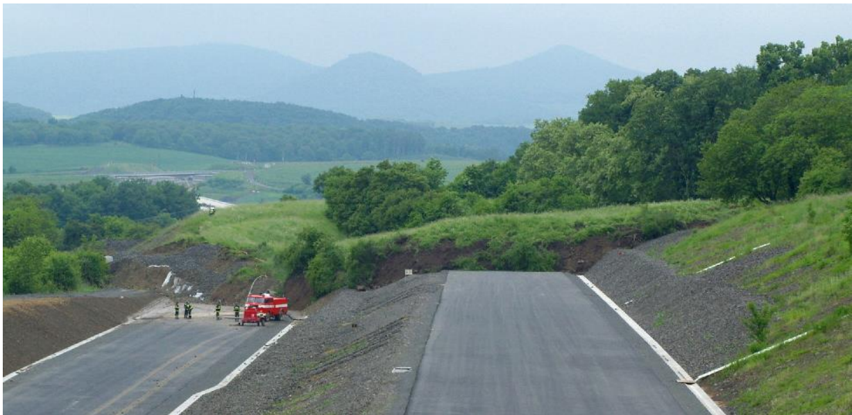
Fig. 1: Damaged motorway D8 which was under construction at the time of landslide.
